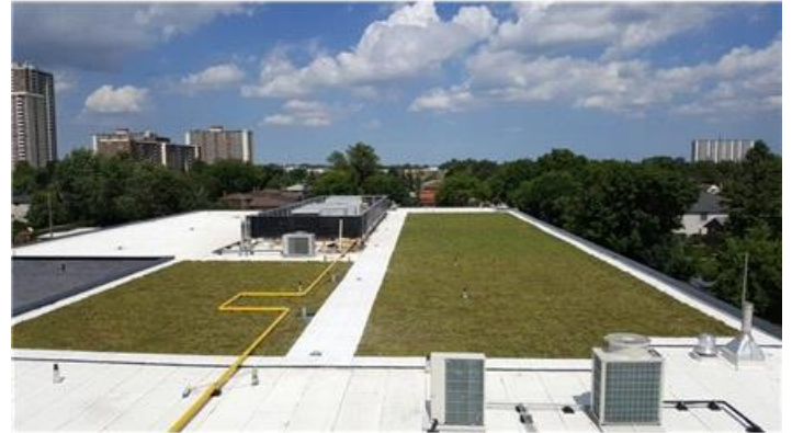
St Paschal Green Roof
